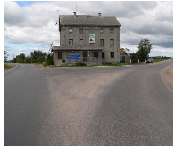
The junction with the road No. 182 (5)
