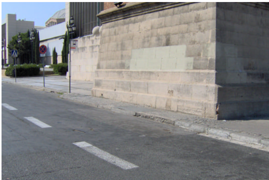
Fig. 6. Width too small of the sidewalk in front of the Venecian towers
