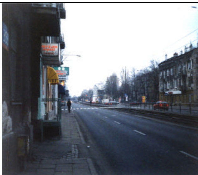
To small width of pavement in the direction of Wiatraczna Roundabout
