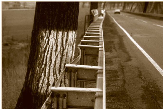
Crash barriers offer protection from roadside objects such as trees
