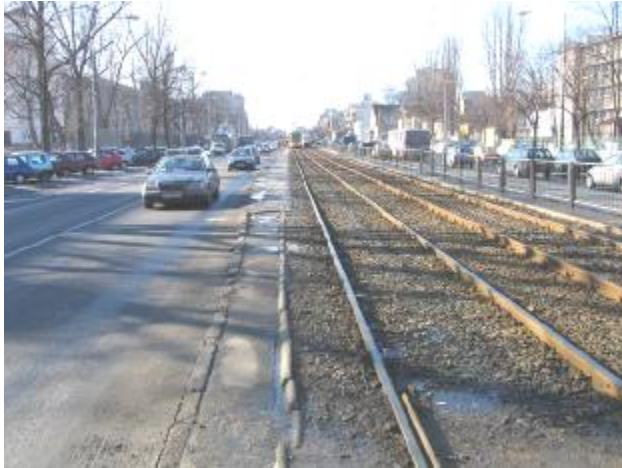
Fot. 3. Grochowska st. – tram track situated in roadway division belt – without refuge for pedestrians crossing the street.
